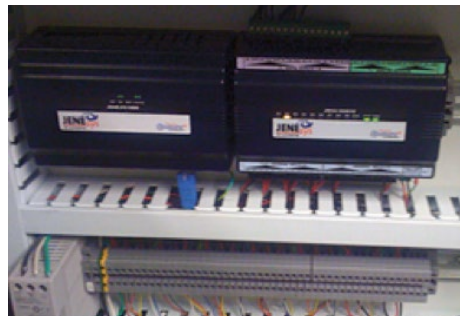
A sensor in the air stream is monitored by the Central Control Unit on the left, which in turn responds to temperature changes to servers in the data center.
