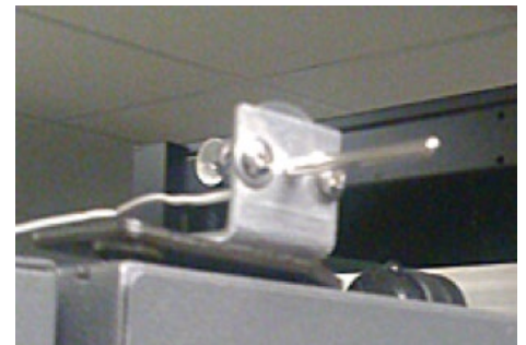
A sensor in the air stream is monitored by the Central Control Unit on the left, which in turn responds to temperature changes to servers in the data center.
